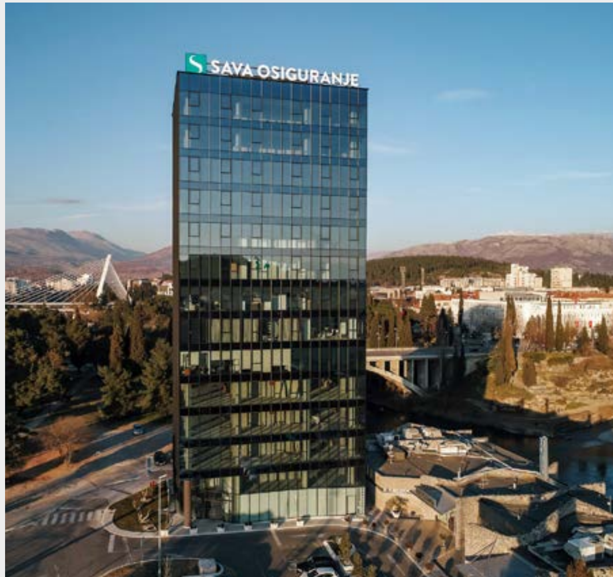
The new business premises in Montenegro boast a new energy-efficient heating and cooling system.
